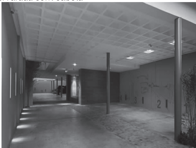
Figura 6 – Laje nervurada com cubeta
